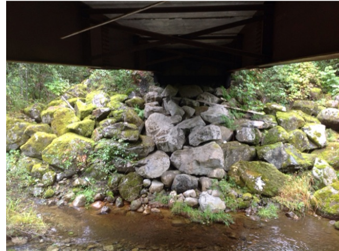
Left Bank Abutment when facing downstream
