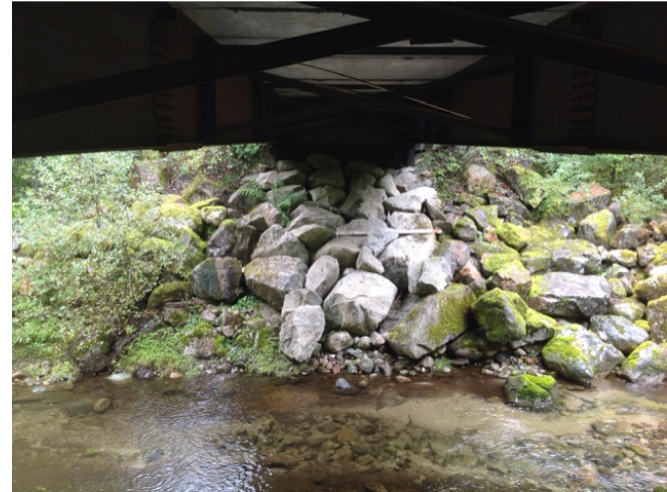
Right Bank Abutment when facing downstream
